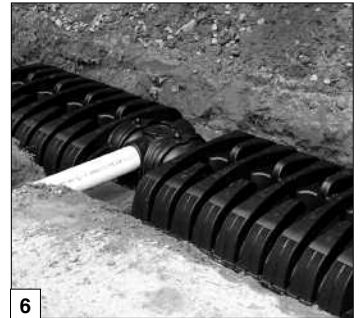
All-in-One as mid-line connection.
