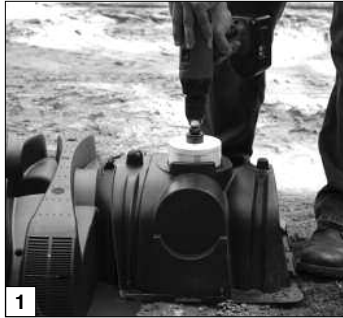
1 Drill Quick4 Plus Periscope.
