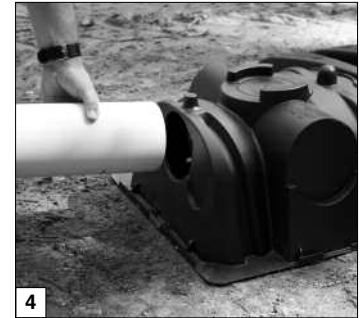
4 Insert inlet pipe.
