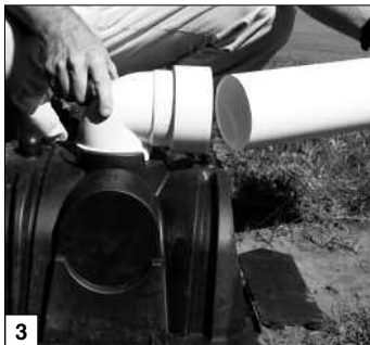
3 Connect inlet pipe.
