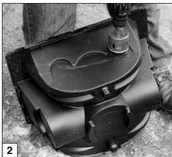
Drill pressure pipe hole.
