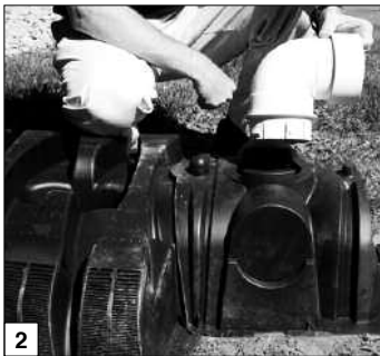
2 Insert Quick4 Plus Periscope.
