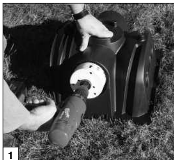
Drill sides or top of All-in-One Endcap.
